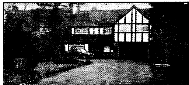
SUBSTANTIAL: Platt's High Barnet home
